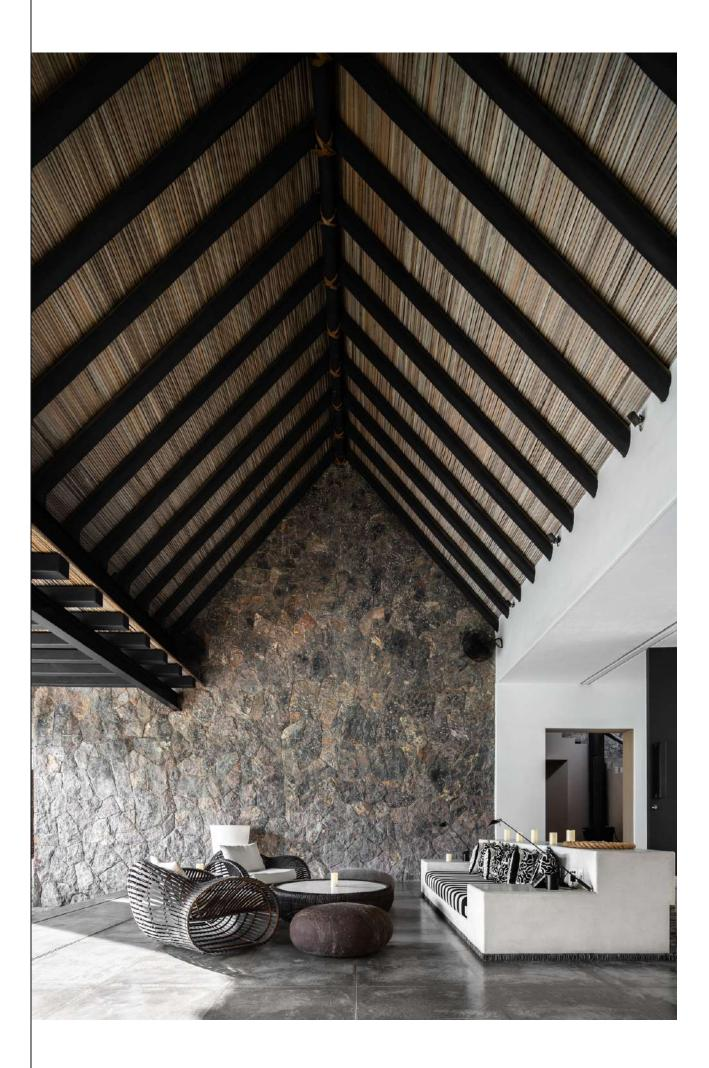
"The use of dry palm for roof construction is an example of sustainable architecture made with recycled materials. In addition, the dry palm is a material that allows the decrease of temperature in hot and tropical environments. Likewise, the stone walls that limit the borders of the house, both exterior and interior, were built with rocks of various sizes and colors taken from nearby rivers, which is also an ideal example of sustainable architecture with reused materials."
